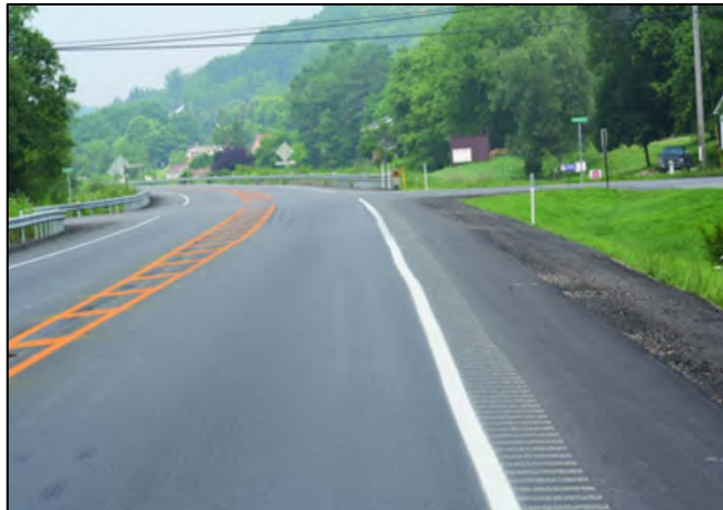
Figure 60. Photo. Pavement markings narrow the travel lane as the driver approaches the intersection.
