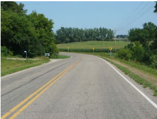
Figure 4. Photo. Delineation with chevrons. Source: MnDOT.
