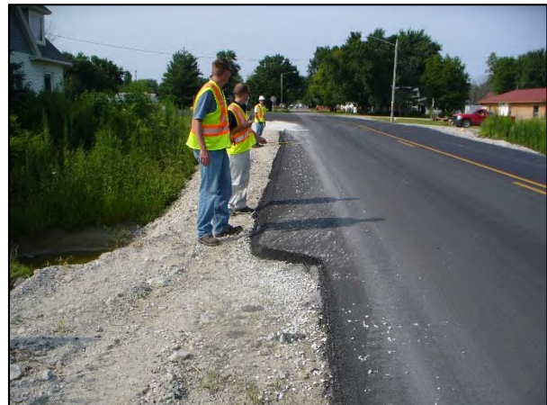
Figure 44. Photo. Shoulder paving operation.
