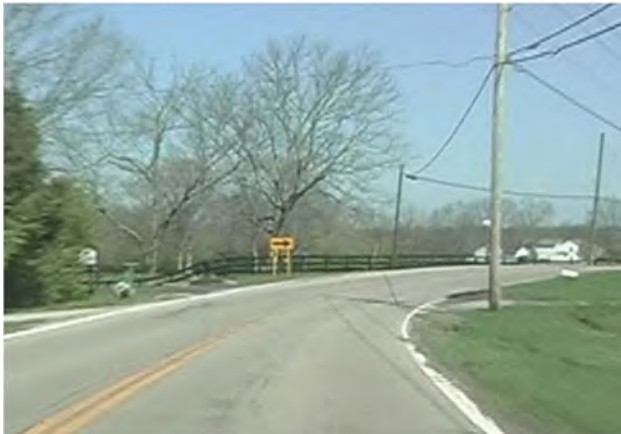
Figure D-3. Photo. A curve on a rural, two-lane road before signage updates through the Horizontal Curve Program.
