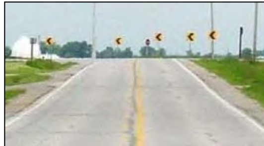
Figure 24. Photo. After, with chevrons. Chevrons provide advanced alignment of a curve.
