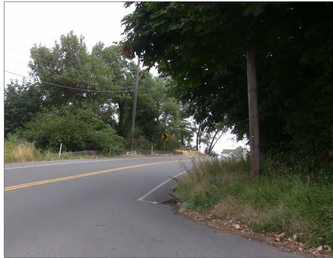
Figure 63. Photo. Sight distance is limited due to the intersection being inside the curve.
