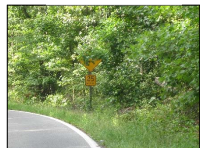
Figure 39. Photo. Curve warning sign covered by foliage.
