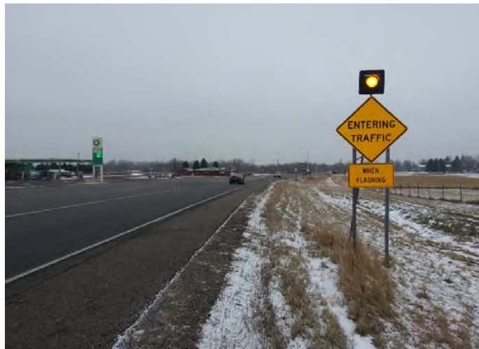
Figure 65. Photo. A dynamic warning sign alerts drivers in real time of other users in the roadway.
