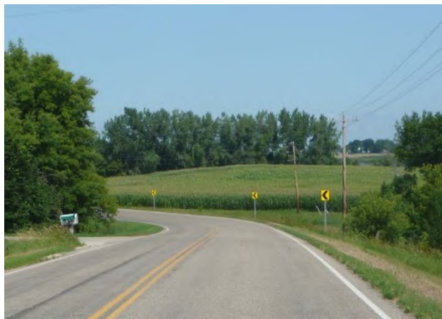
Figure B-2. Photo. MnDOT installed chevrons as part of their Systemic Safety Improvements Program.
