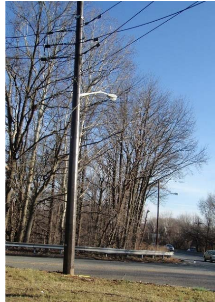
Figure H-2. Photo. NJDOT used utility poles made from fiberglass that would collapse upon impact and not break away into the road.
