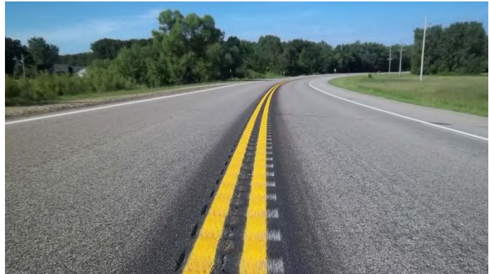
Figure 5. Photo. Centerline rumble strips.
