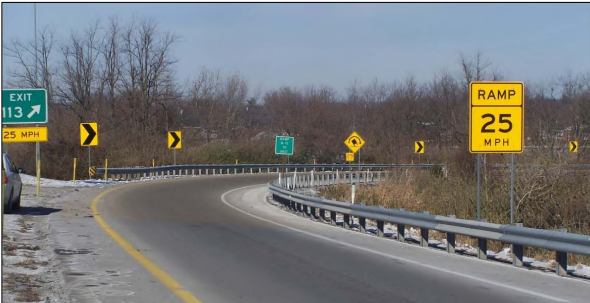
Figure 52. Photo. Barrier along inside and outside of horizontal curve.
