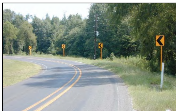
Figure 25. Photo. Chevrons assist the driver in navigating curves. Source: Texas Transportation Institute.
