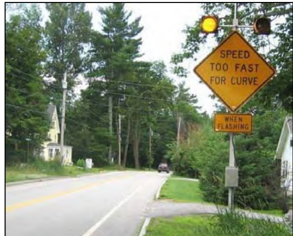
Figure 33. Photo. Flashing Beacon on Warning Sign, Augusta, ME.
