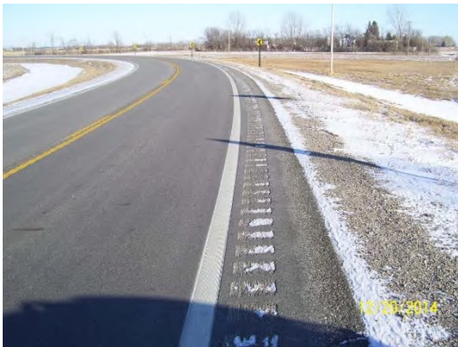
Figure 6. Photo. Adding narrow paved shoulders (2 feet) to existing top width. Includes rumble strips and Safety Edge SM . Source: MnDOT.
