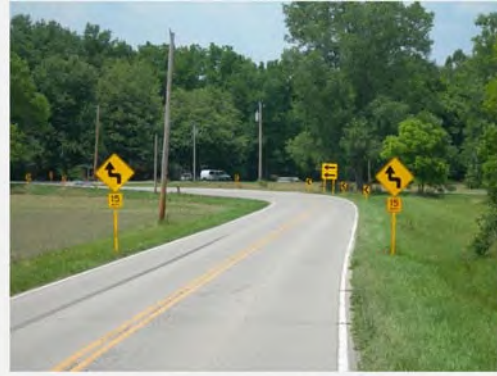
Figure 28. Photo. After signage updates.
