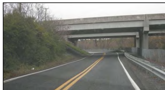
Figure 9. Photo. Edge lines.
