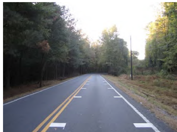
Figure 15. Photo. Optical speed bars are designed to reduce vehicle speed. Source: KLS Engineering.
