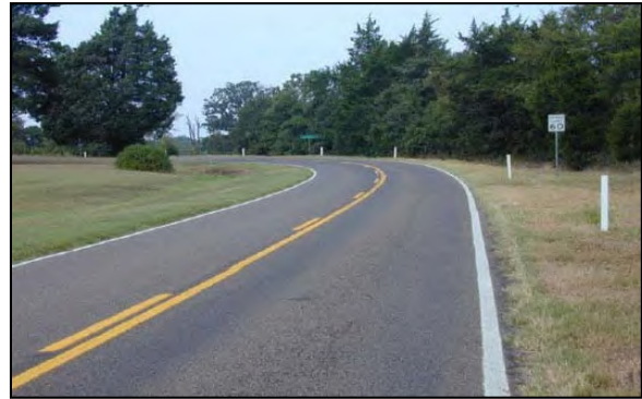
Figure 12. Photo. The color of delineators must match the color of the adjacent edge line. Source: Texas Transportation Institute.
