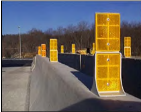
Figure 57. Photo. Delineated concrete barriers. Source: Michigan DOT.
