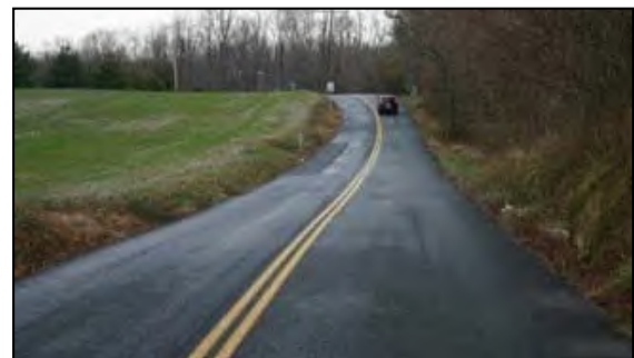
Figure 8. Photo. Center line for No Passing on horizontal curve.
