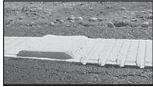
Figure 18. Photo. An example of profiled pavement markings. Source: Caltrans.
