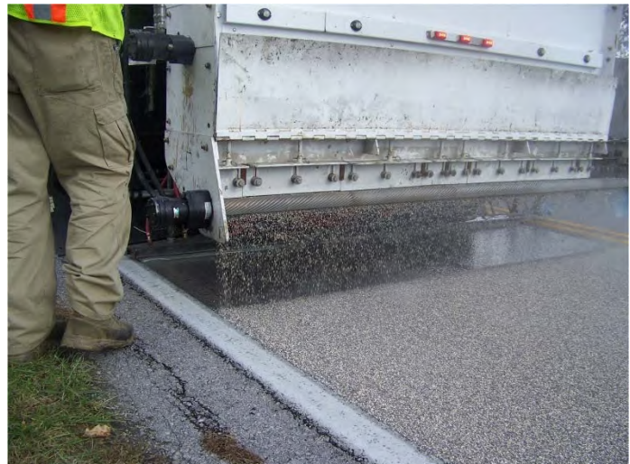
Figure F-1. Photo. A truck in the process of applying HFST to a curve.
