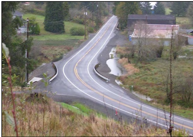
Figure 67. Photo. Intersection with paved approach.
