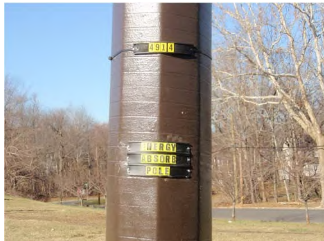
Figure H-1. Photo. A close-up of the energy absorbing utility poles used as a part of NJDOT's pilot project.
