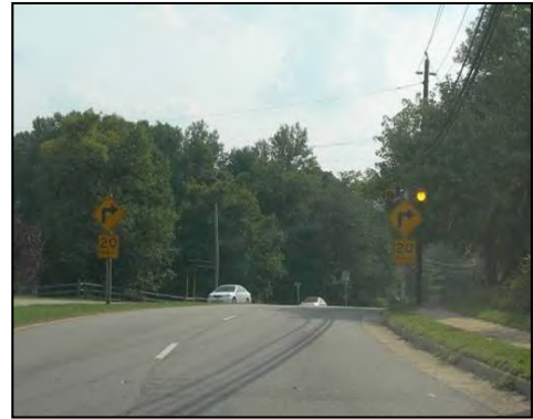
Figure 31. Photo. Typical arrangement of signs and flashing beacons.
