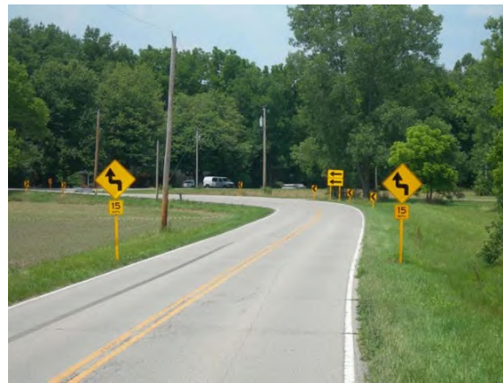
Figure D-2. Photo. A curve on a rural, two-lane road after signage updates through the Horizontal Curve Program.
