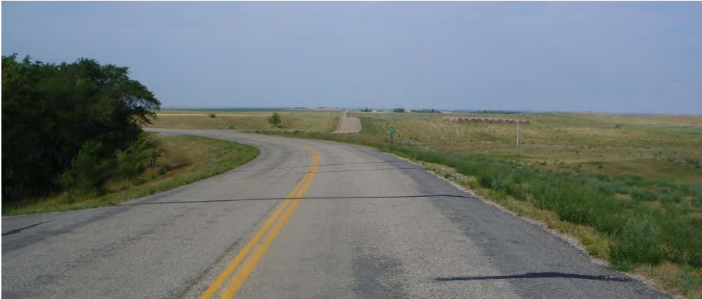
Figure 62. Photo. An example of a visual trap exists when a crest vertical curve blocks the view of the upcoming horizontal curve (top photo). What appears to be a continuation of the road in the distance is actually an intersecting roadway in the midst of a curve (bottom photo).
