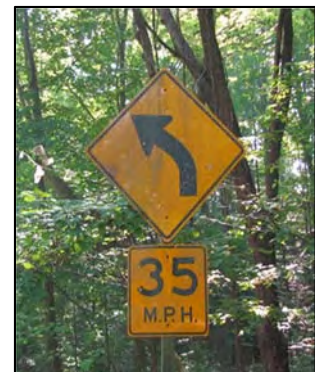
Figure 38. Photo. Low Retroreflectivity sign example.
